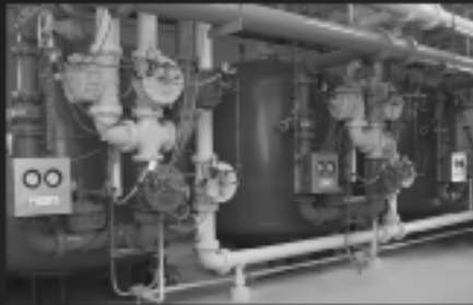
Radium and Iron Removal Systems
