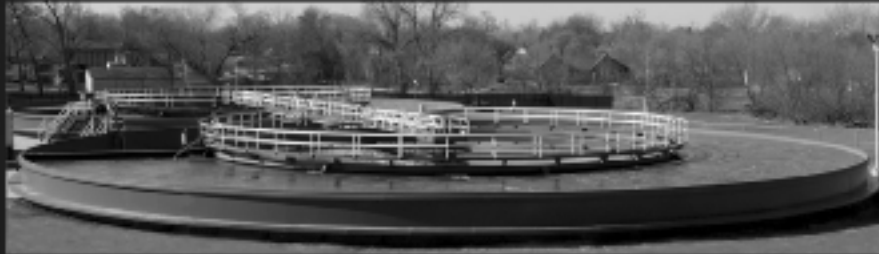
Wastewater Treatment Solutions
