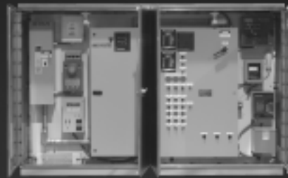
Pad Mounted Control Packages
